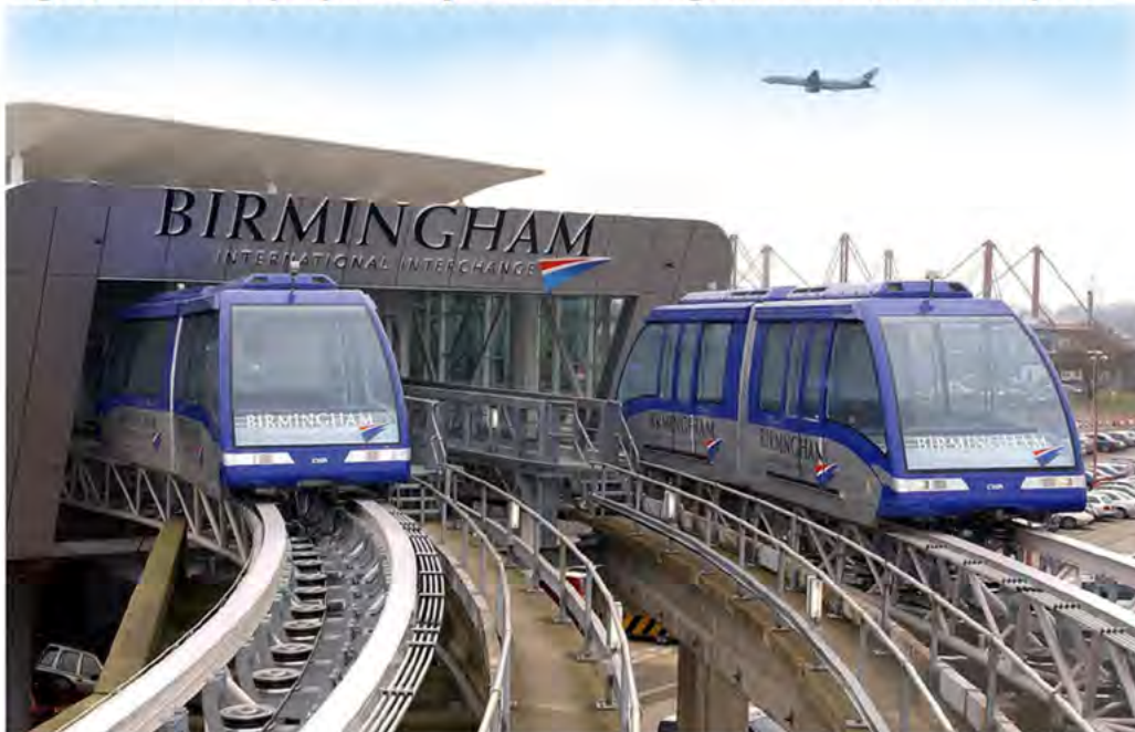
Figure 31: Cable-propelled system at Birmingham International Airport 7
