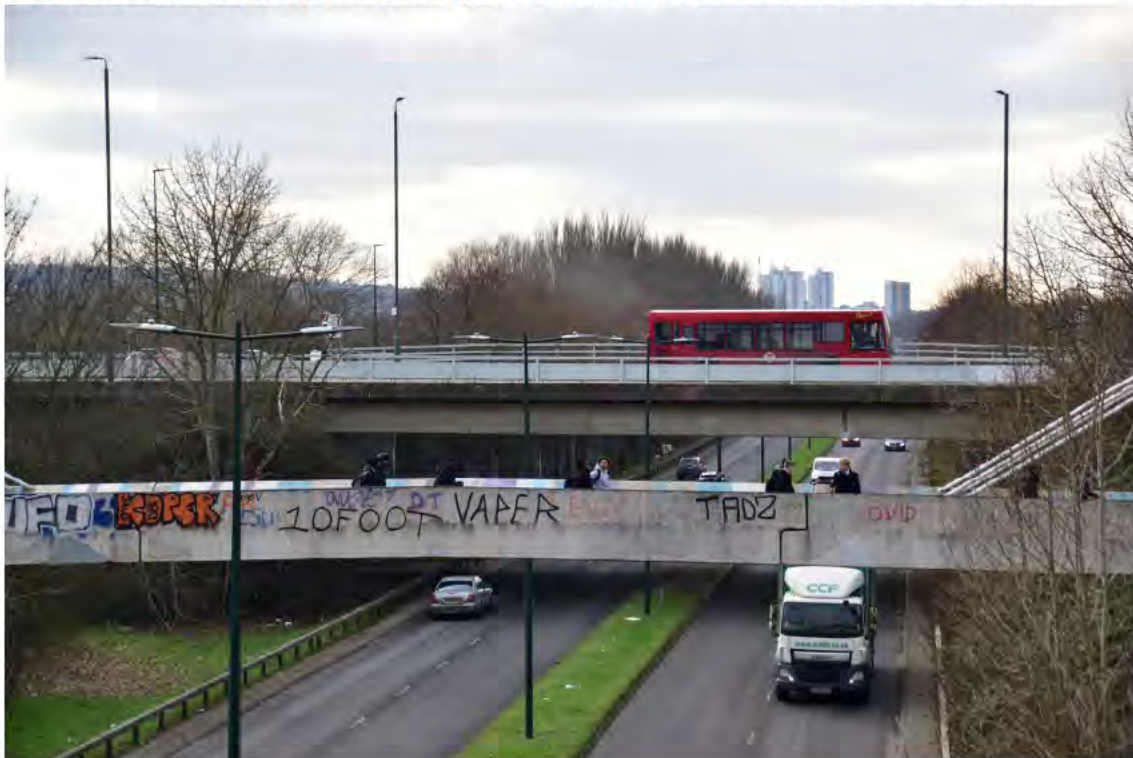
Figure 47: Existing highway and pedestrian infrastructure in Thamesmead
