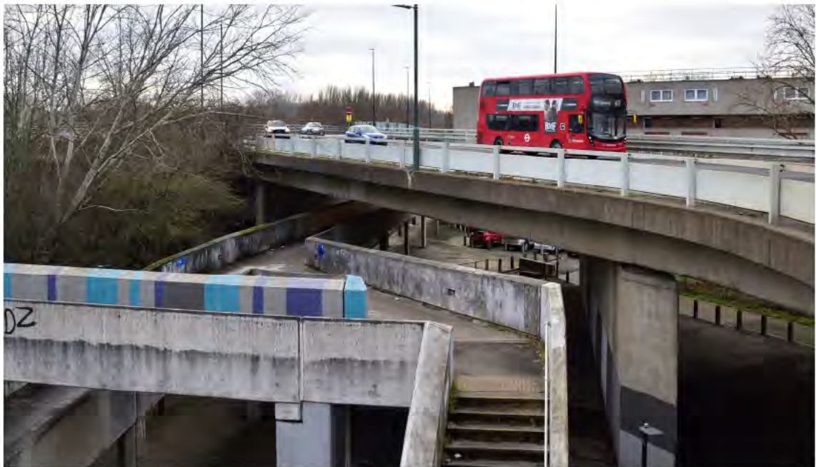
Figure 9: Pedestrian/cycle bridge linking Thamesmead to Abbey Wood
